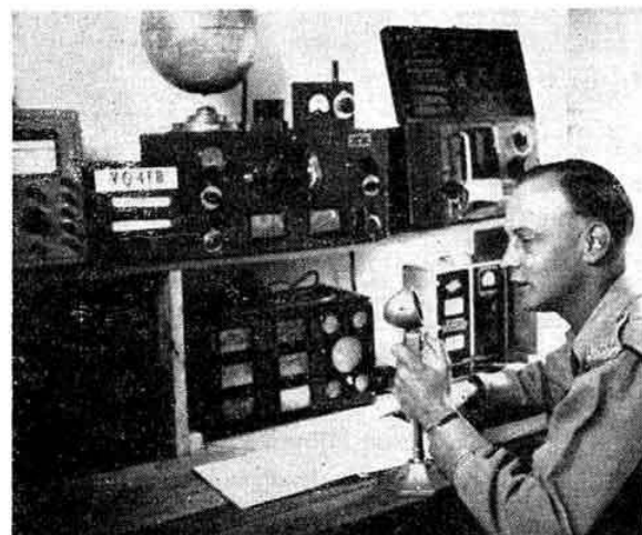
VQ4FB is operated by Fred Ward (ex-G3CAT and VU2AT) from a site 5000 ft. a.s.l. at Meru, Kenya. The transmitter is a B2 and the receiver an HRO. A 67 ft. "V51AA" aerial is used on all bands from 3.5 to 28 Mc/s. Listener reports (which are welcomed) and QSL cards may be sent to Box 1313, Nairobi (the QSL Bureau) or direct to the Signals Officer, Kenya Police Div. H.Q., Meru, Kenya.
